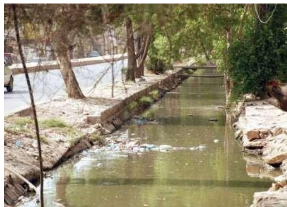
Fig: 3. Water channel (Wadhu Wah) Qaimabad
