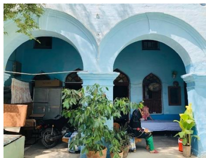
Fig 3: Existing verandah in vernacular building of Hirabad
