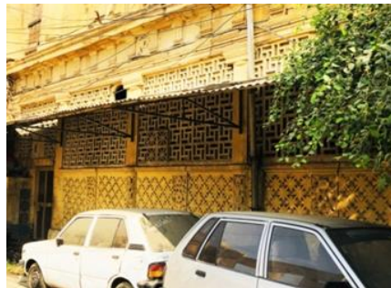
Fig 5: Mashrabiya in an old building of Hyderabad to provide natural ventilation and privacy.
