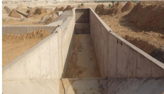
Fig. 4: Stilling Basin at Darawat Dam
