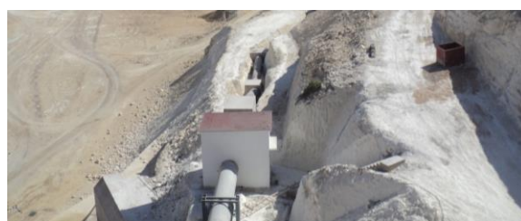
Fig. 3: Irrigation Conduit at Darawat Dam
