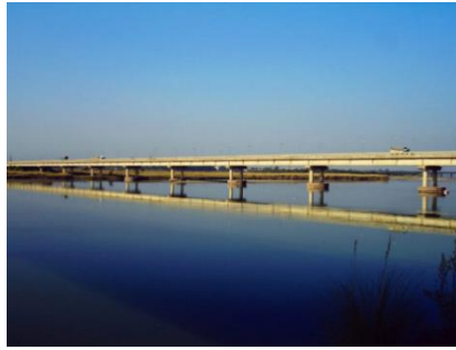
Fig. 2: Bridge on river Sutlej, Pakistan having circular compound bridge piers.
