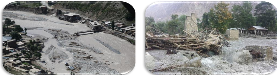
Fig 1: Bridge collapse during 2010 flood on river swat
