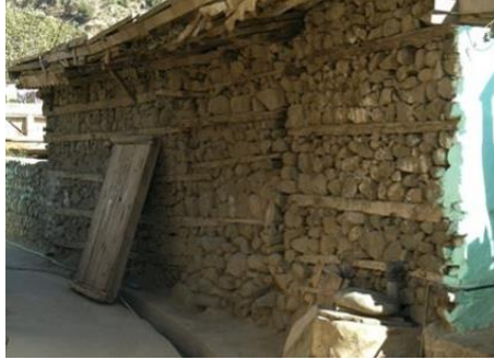
Fig. 5: Bhattar construction in Northern Pakistan Photo by: Randolph Langenbach
