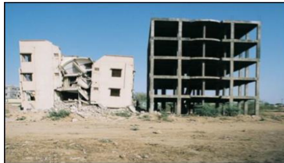
Fig. 3: Buildings in India that were meant to be identical.
