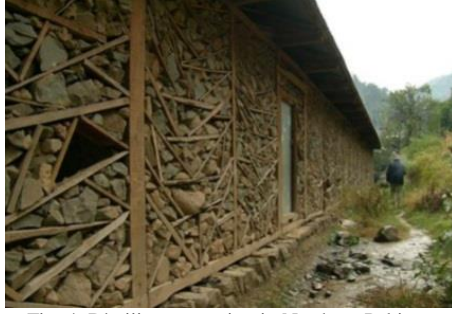
Fig. 4: Dhajji construction in Northern Pakistan Photo by: Randolph Langenbach
