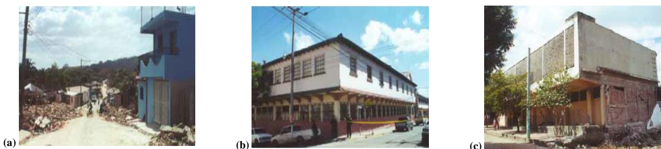
Fig. 6: Behavior of confined masonry during the 2001 El Salvador earthquakes, (a) confined masonry structures in city of Santa Cruz Analquito survived, whereas nearby conventional structures was destroyed, (b) a confined masonry school building survived the earthquake without damage (c) soft story construction (confined masonry construction at the ground floor level) [36]
