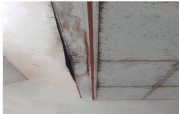
Figure 13: Wall Finishes peeling due to water seepage, Source; Author's Fieldwork 2019
