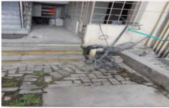
Figure 10: Damaged Pavers of Apartment Building, Source; Author's Fieldwork 2019
