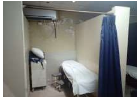
Figure 13: Wall Finishes peeling due to water seepage, Source; Author's Fieldwork 2019
