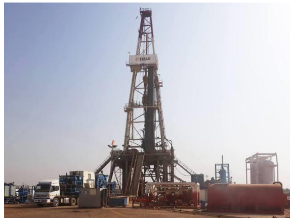
Fig. 1: drilling rig bentonite mud using during drilling process
