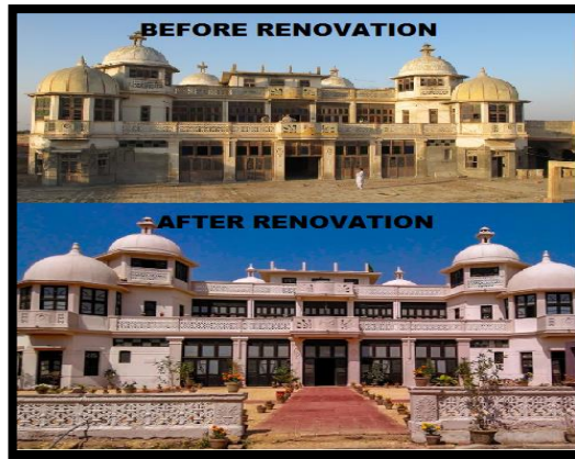
Fig. 7: Architectural condition before and after renovation of “Sahib Mahal Badin”
