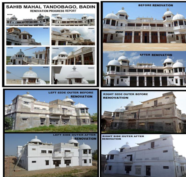
Fig.5: Exterior views before and after renovation of “Sahib Mahal Badin”
