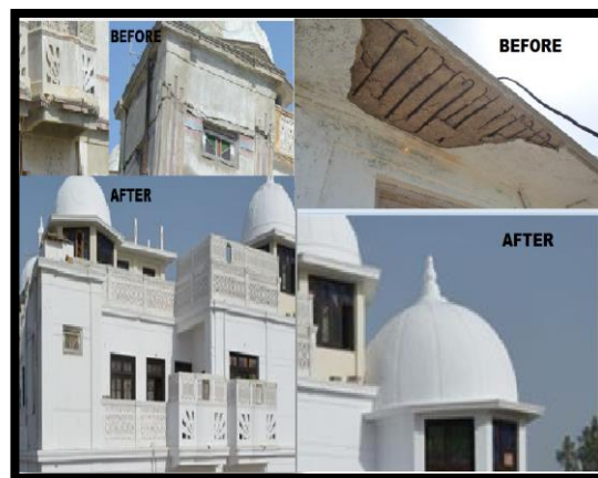
Fig. 6: Views of structural renovation of “Sahib Mahal Badin”
